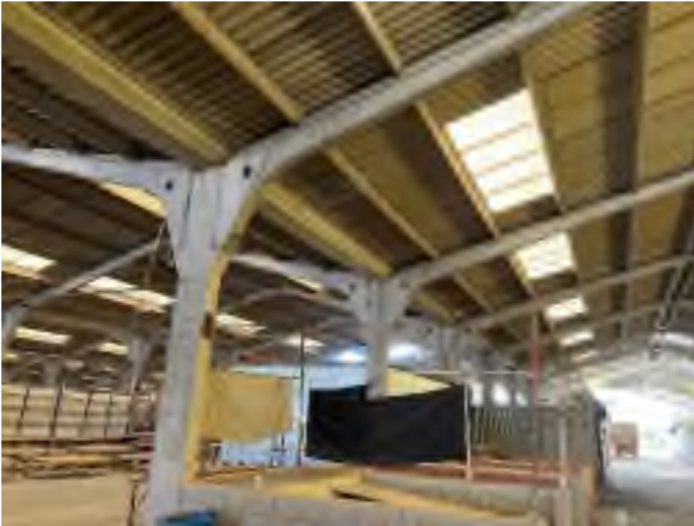
An Inside View of the Rooftop
