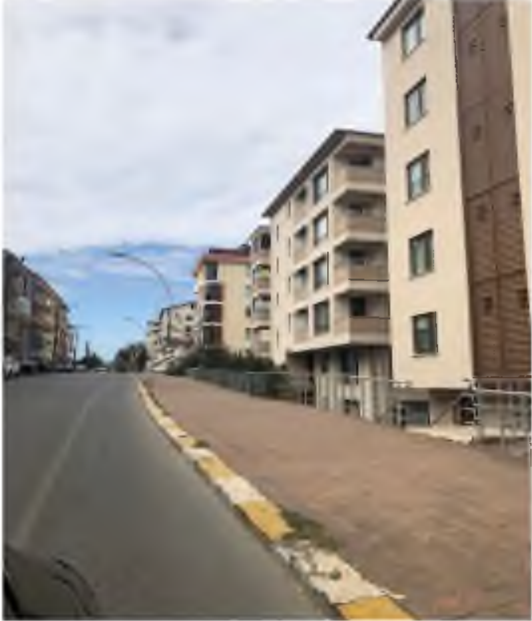
General View İstanbul Avenue
